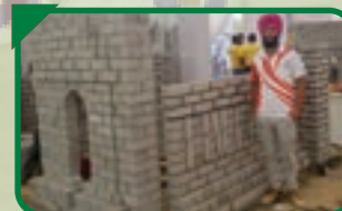
Roop Singh Student of Engineering participated at National Skill Competitions in Brick laying organized by Skills India for World Skills Competition in Russia
